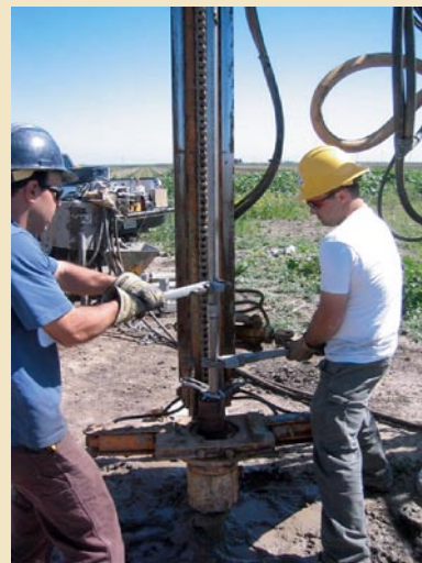
Installing deep drill GPS requires continual adjustments to the rig and bit while it drills 30 ft below ground.
