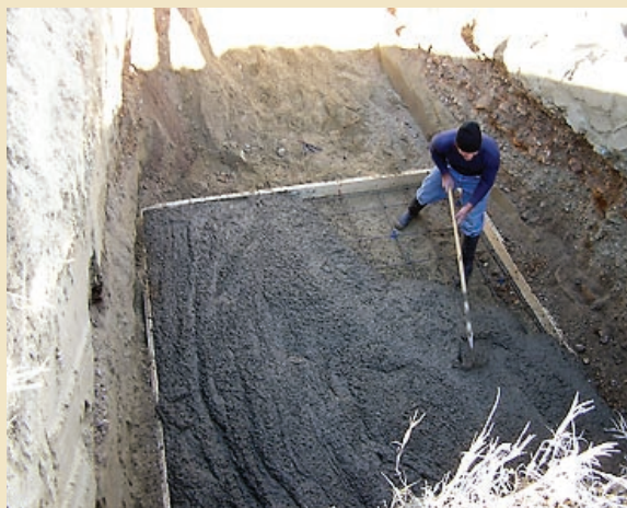
J. Anderson spreading concrete for the ANSS Backbone slab in Dagmar, Montana.
