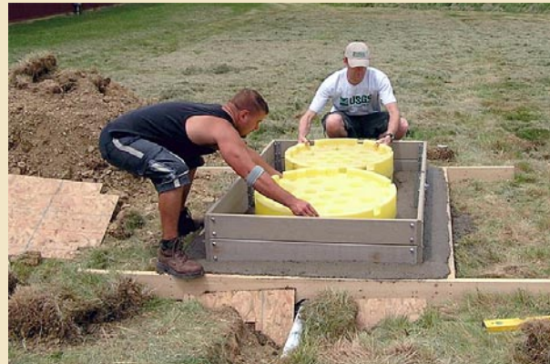
J. Anderson and J. Fox setting the McMillan Vault enclosure at ACSO (Alum Creek State Park, OH).
