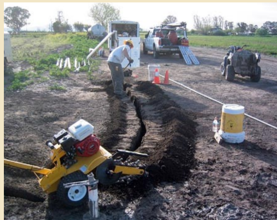
Cable and conduit are laid below ground to connect the enclosure with the GPS monument.
