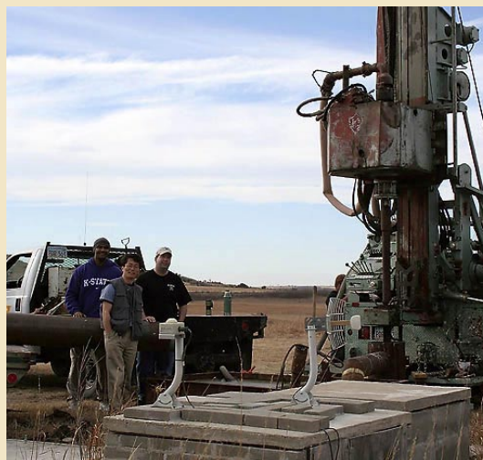
Drilling the seismic vault in Kansas.
