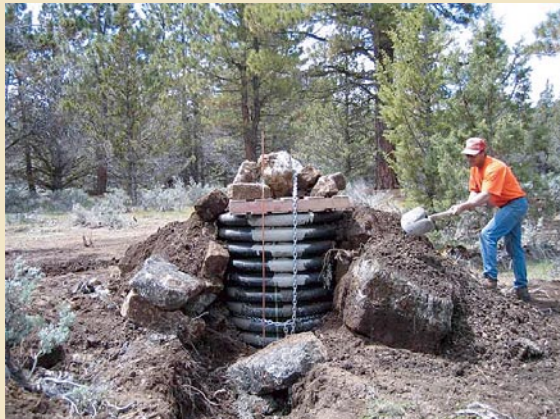
S. Christman adds thermal and environmental protection around the ELFS (Eagle Lake, CA) vault. The vault could not be completely buried due to a thin soil layer (0.7 m) over very hard basalt basement.
