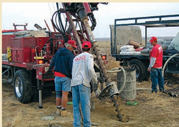
Drilling for Utica Cal Trans GPS station P547 in Southern CA.
