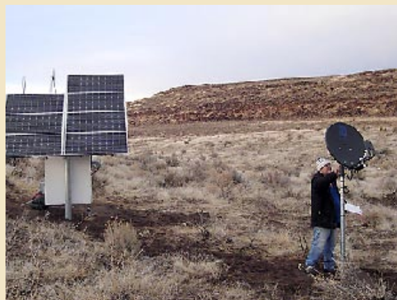
K. Oliver installing a VSAT system at the Transportable Array station in Valley Falls, Oregon.
