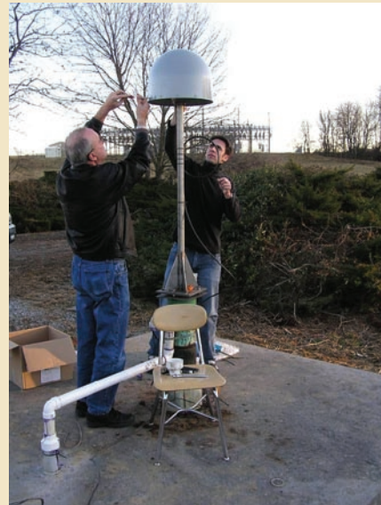
Installing the custom GPS monument at the ANSS Backbone site in Blacksburg, VA.
