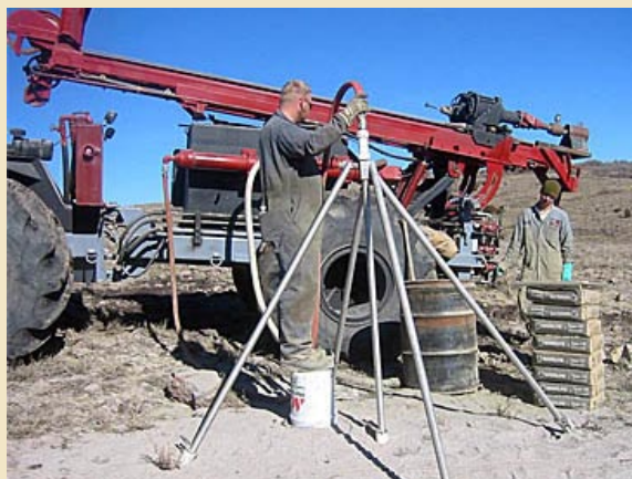
Pumping cement into the long legs of a deep drill GPS station in Northern Wasatch County, Utah.
