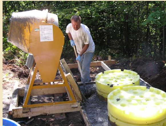
Constructing a surface seismic vault for the ANSS Backbone station near Lake Ozonia, NY.
