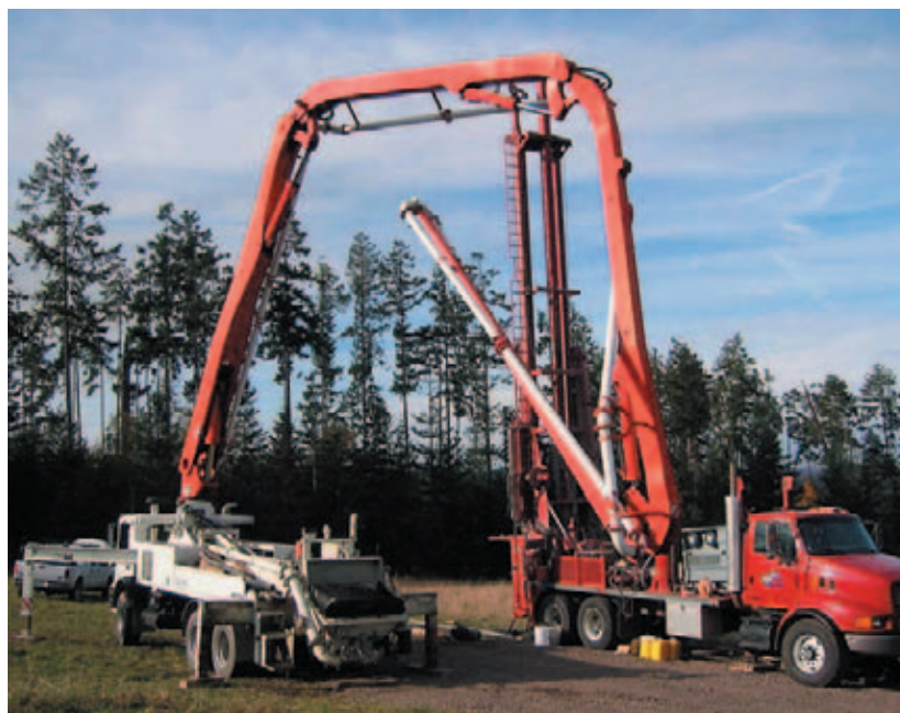
Cement pump truck at an Olympic Peninsula strainmeter borehole.
