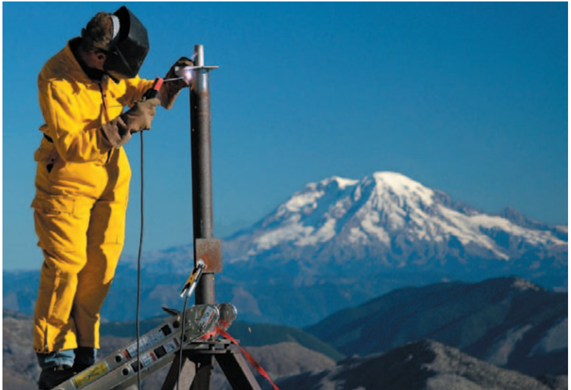
PNW Field Engineer Peter Gray welding the antenna base on to an EDM tower at P695 (Nelson Ridge, MSH).
