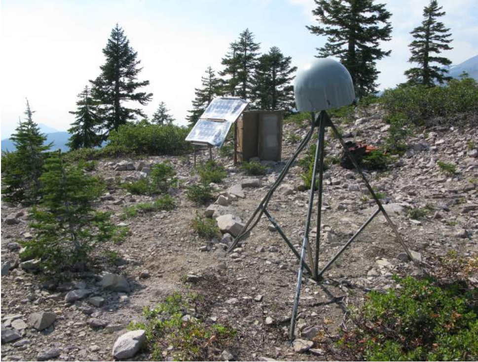
Overview photo of station P656 on the slopes of Mount Shasta, taken by a UNAVCO field engineer during a visit to repair the station after it had gone offline due to heavy snow. Note the damaged solar panel and the broken radome. This station was likely buried under several meters of snow.
