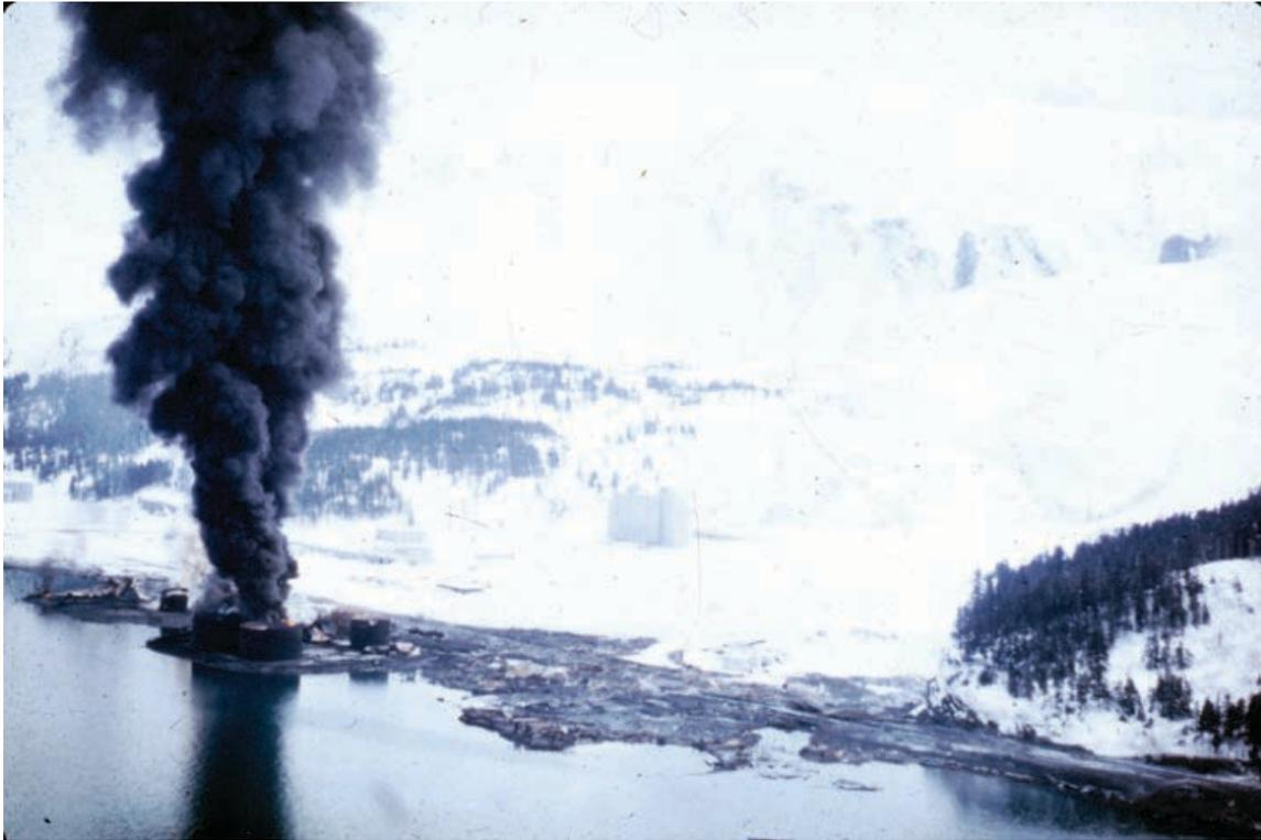
*Figure 8.1. Alaska Earthquake March 27, 1964. The dock area, a tank farm, and railroad facilities at Whittier were severely damaged by surge-waves developed by underwater landslides in Passage Canal. The waves inundated the area of darkened ground, where the snow was soiled or removed by the waves (USGS).*
