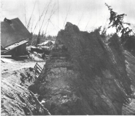
*Figures 2.3. Top: Sketch section through eastern part of Turnagain Heights slide. Note pressure ridge, upright blocks at center and to left of pressure ridge, and tilted collapsed blocks between (from Hansen, 1966). Bottom: Photo taken from within Turnagain Heights slide. Sharp-crested clay ridge, with collapsed blocks tilted toward ridge on both flanks. Note horizontal stratification in ridge.*
