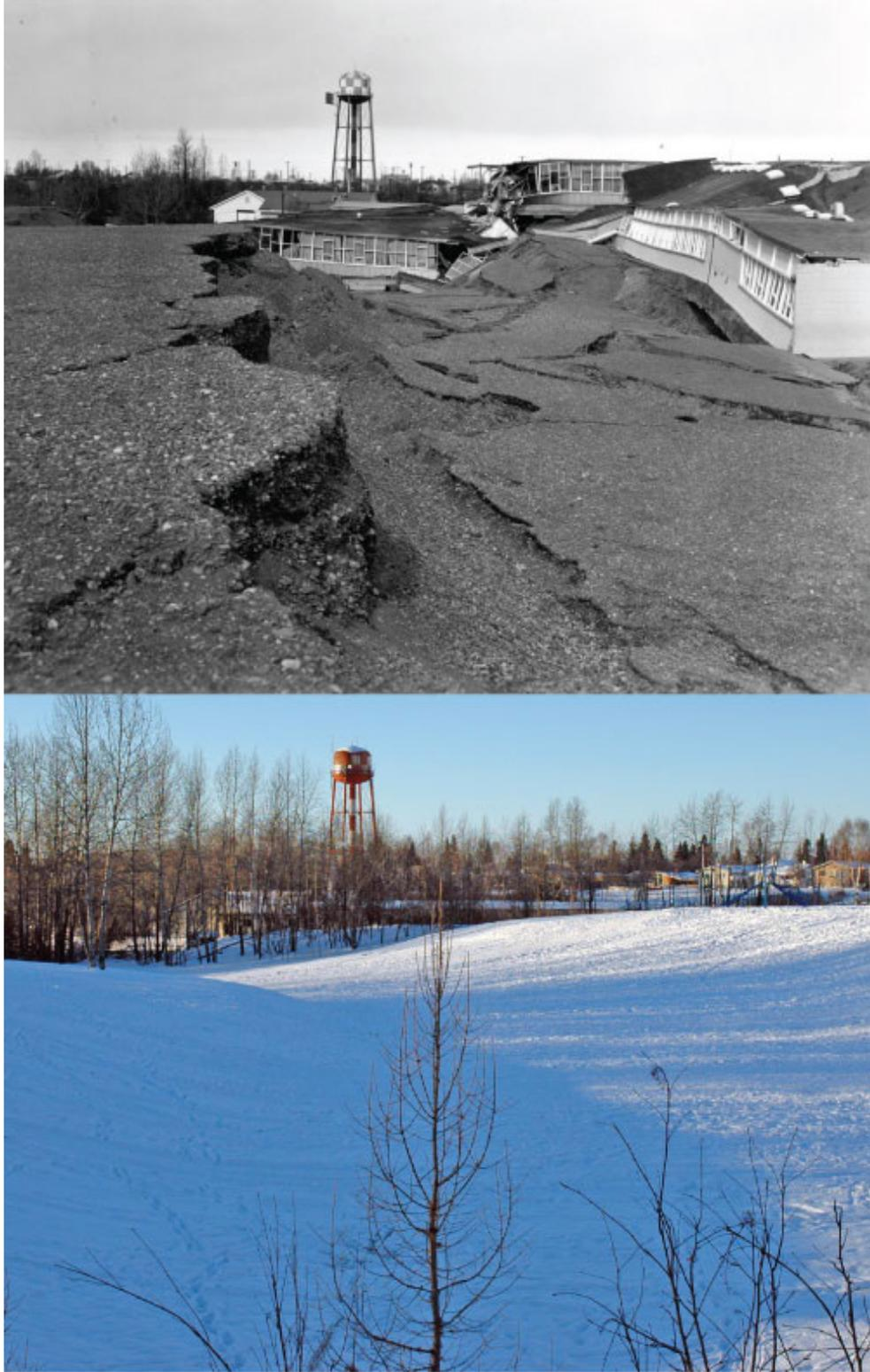
*Figure 1.2. Top: View to the west showing the Government Hill School collapsed into a graben, or linear trough, formed by the Government Hill landslide in 1964. Bottom: Same view in 2013 (photo: Game McGimsey). The graben formed by the landslide is still expressed in the landscape in the lower photo.*
