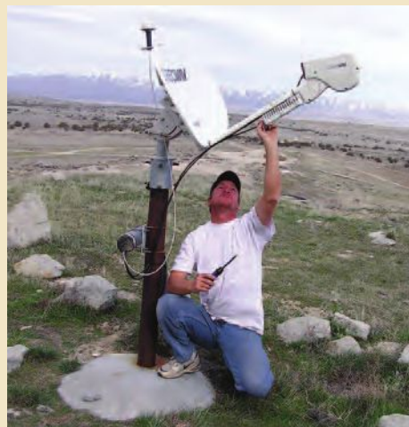
S. Roberts adjusts VSAT antenna at ANSS Backbone station near Dugway, UT.
