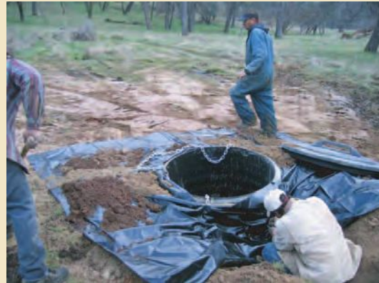
Mitigating against water intrusion at a Transportable Array station using a thick pond liner as a water barrier.
