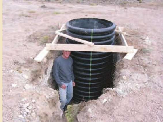
Transportable Array style vault at the Albuquerque Seismological Laboratory for comparison tests with the standard MacMillan design used with the National Seismic Network station upgrades
