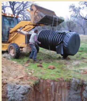
A plastic liner was added to Transportable Array vaults to avoid flooding from California's unusually wet winter.
