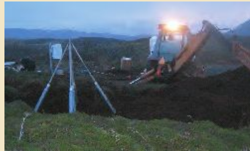
Installation of hybrid deep-short drilled braced monument in Sand Point Alaska.
