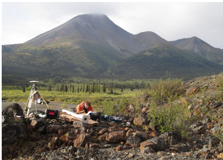
Max Kaufman, Research Assistant with University of Alaska Fairbanks, gets ready to install a continuous GPS station at Macmillan Pass, near the Yukon Territory-Northwest Territories border. Photo by Derek Schutt.
